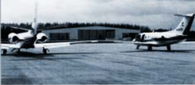
Aircraft cluster around newly completed Weatherwise hangar
